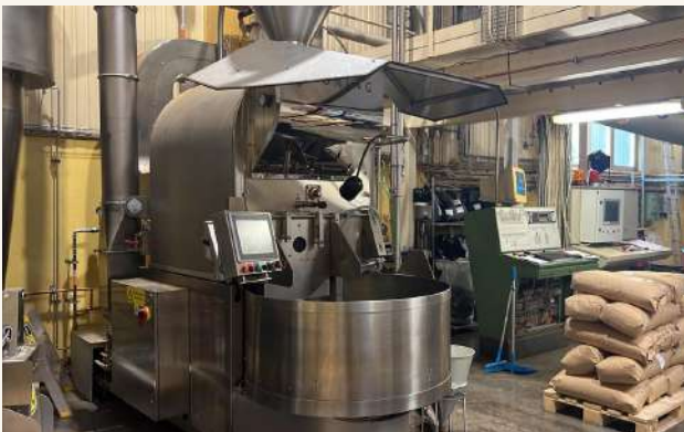
Part of the roasting facility in Gothenburg.
